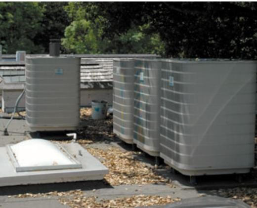
Westinghouse 16 SEER condensing units positioned on the rooftop. Two-speed operation stages the cooling based on need.
